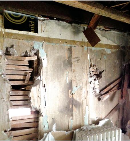
Extensive wall damage (interior and exterior) to a storage room on the 2nd floor of the home.
